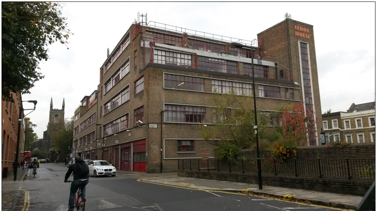
Photograph 3: existing building (Henshall Street and Dove Road elevations, with St Paul's Church in the background)
